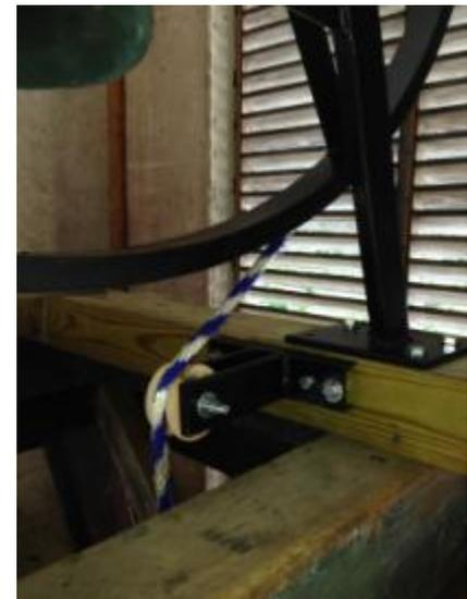
New pulley to help guide “pealing” rope and reduce wear.
